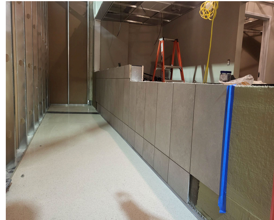
Wall tile installation
