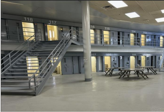
Completed blitz unit
