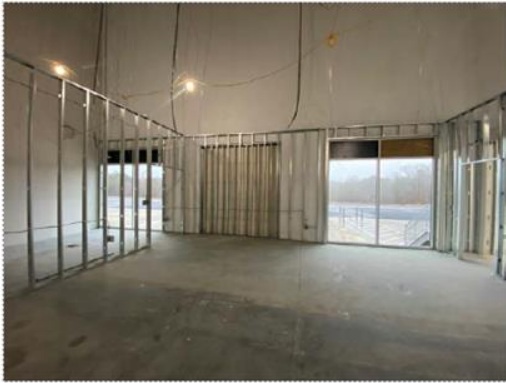
DREAM Office area wall framing commenced
