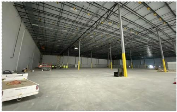
Elections warehouse view looking at Phase 2 demising wall
