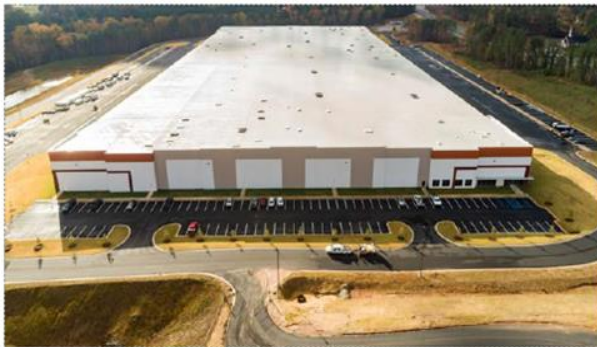
Building west facade
