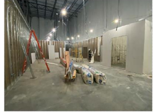
EMA Office Area wall framing
