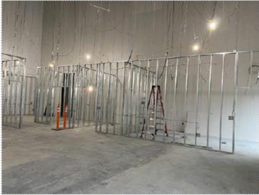
DREAM Office area wall framing
