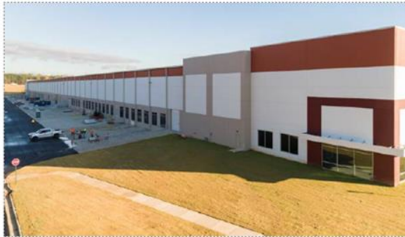
Building south facade
