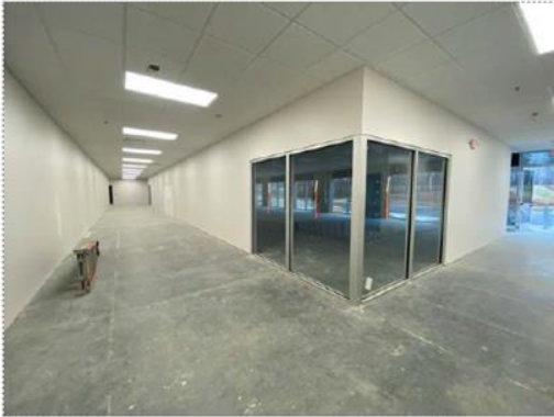
Corner Administration office view at corridor
