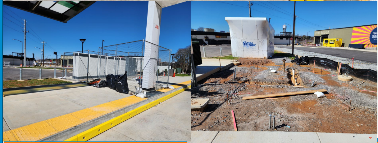
Carver Station – Construction Activities
