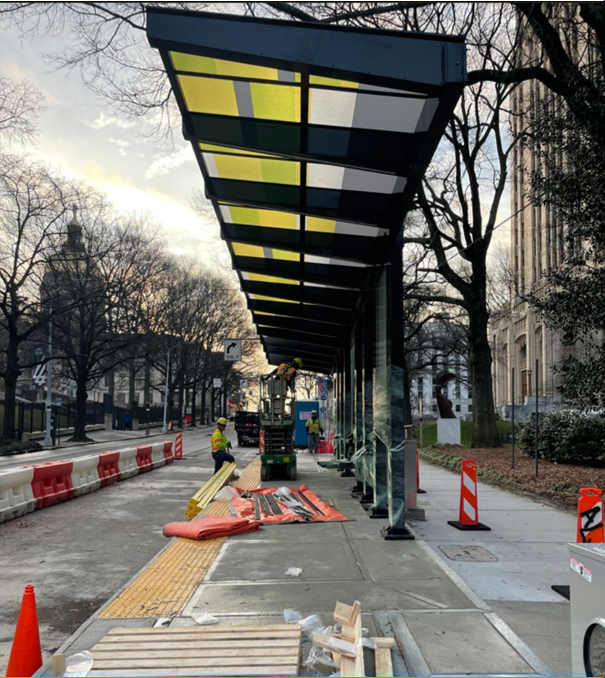
City Hall Station - Shelter Construction
