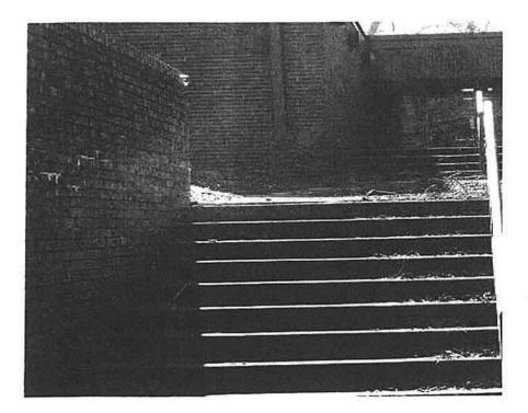
Dirt build-up and mortar repair required on exterior retaining wall
