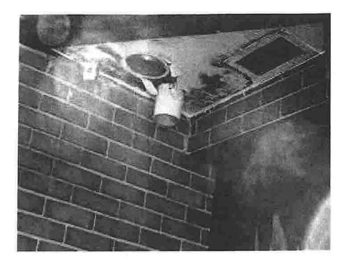
Light fixture damaged and signs of water leaks from roof
