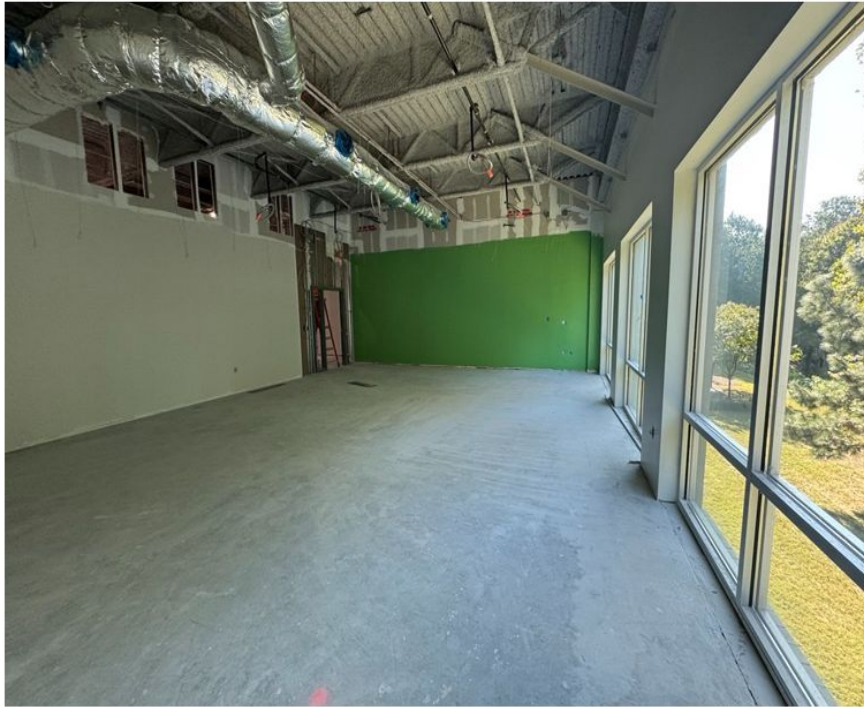
Prime complete and 1 st coat of paint applied.
