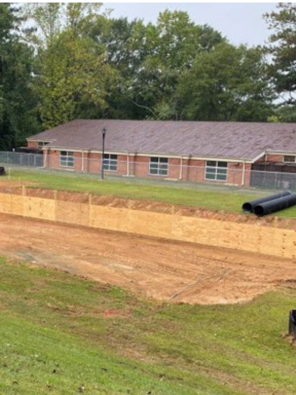
Retention Pond In Progress As of 10/6/2023
