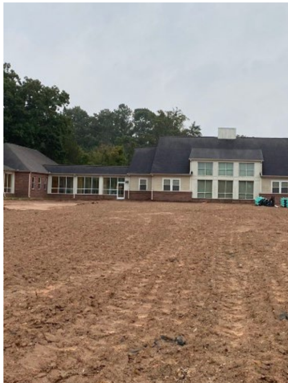
Grading In Progress As of 10/13/2023
