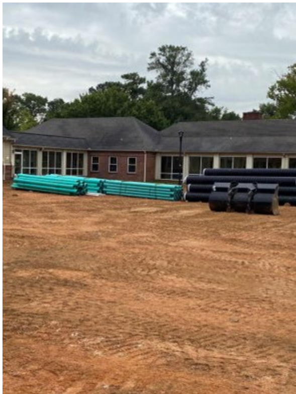
Grading In Progress As of 10/6/2023
