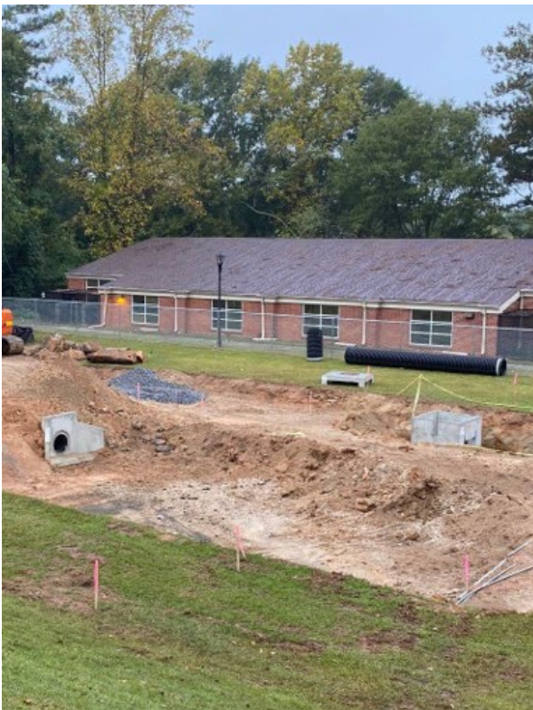
Retention Pond In Progress As of 10/13/2023
