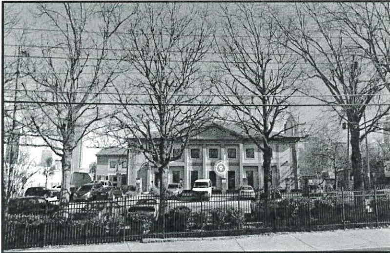
Existing administrative offices
