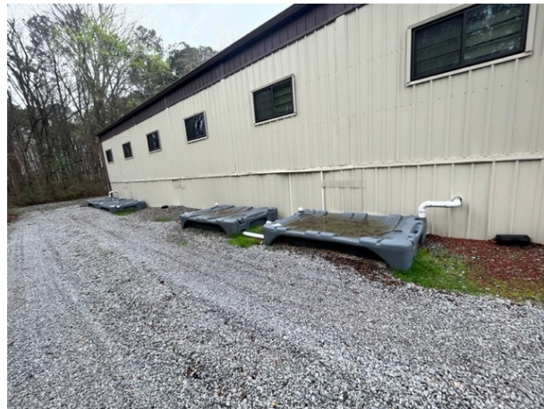
34 : View of aboveground septic tanks located in the rear of the office trailer.
