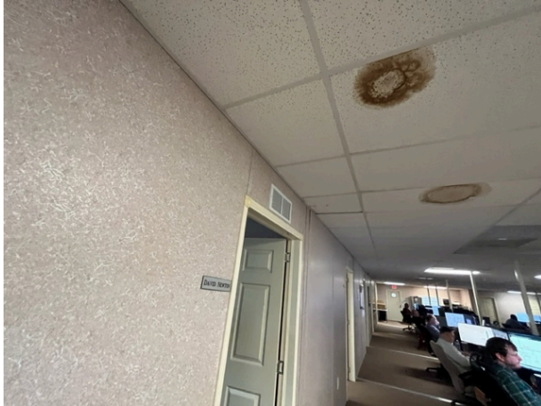
31 : Water damaged ceiling tiles located within the office trailer.
