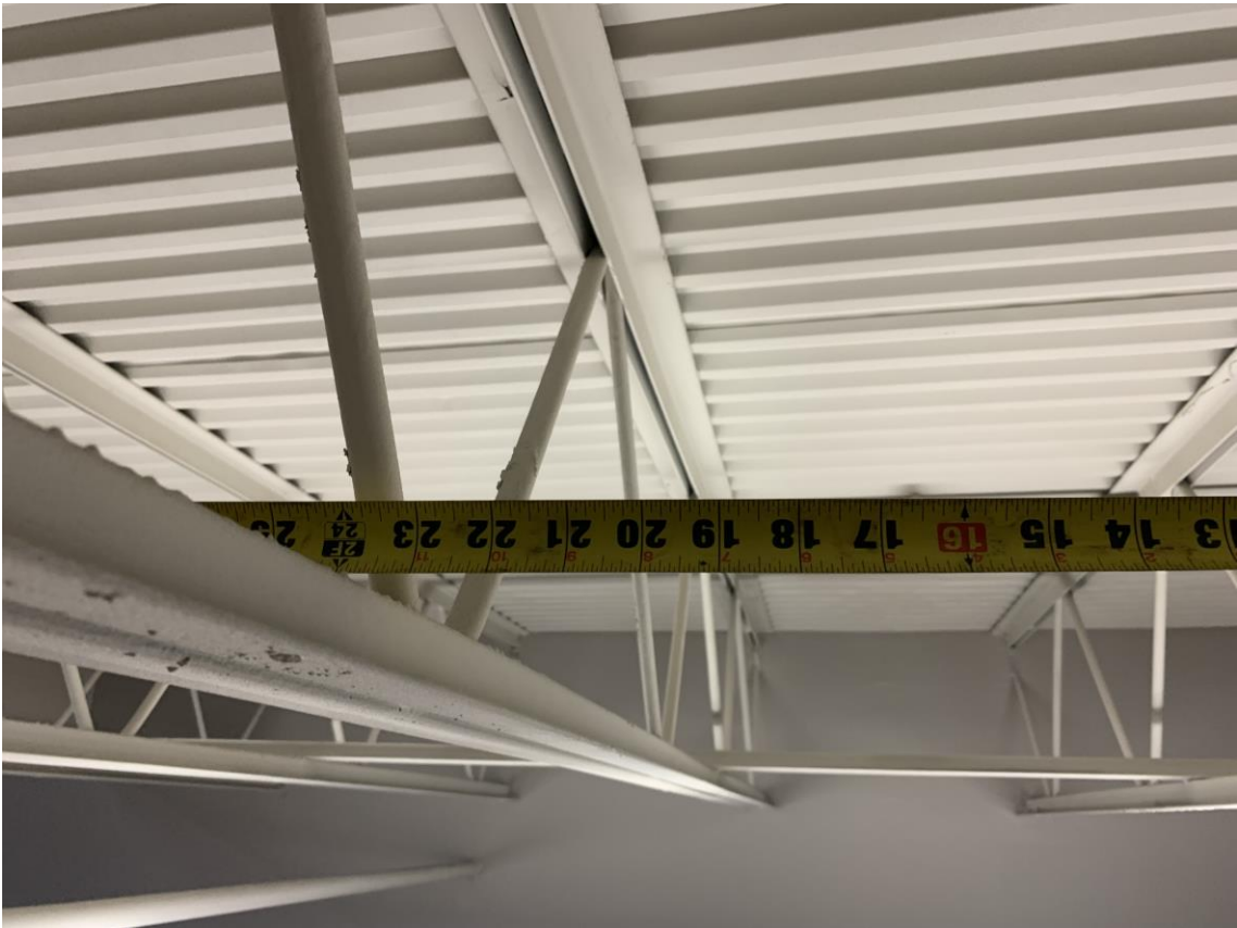
Photos 5 + 6: Spacing of Joists
