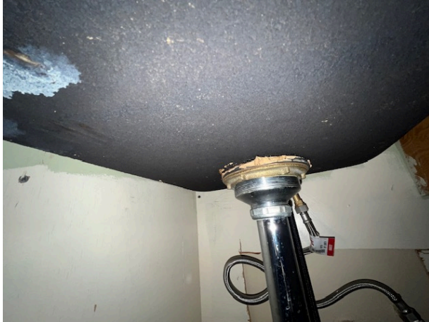
61 : View of positive ACM located under hallway sink within the office building.
