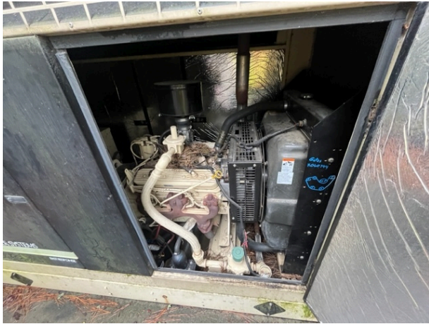
51 : Interior view of emergency generator.
