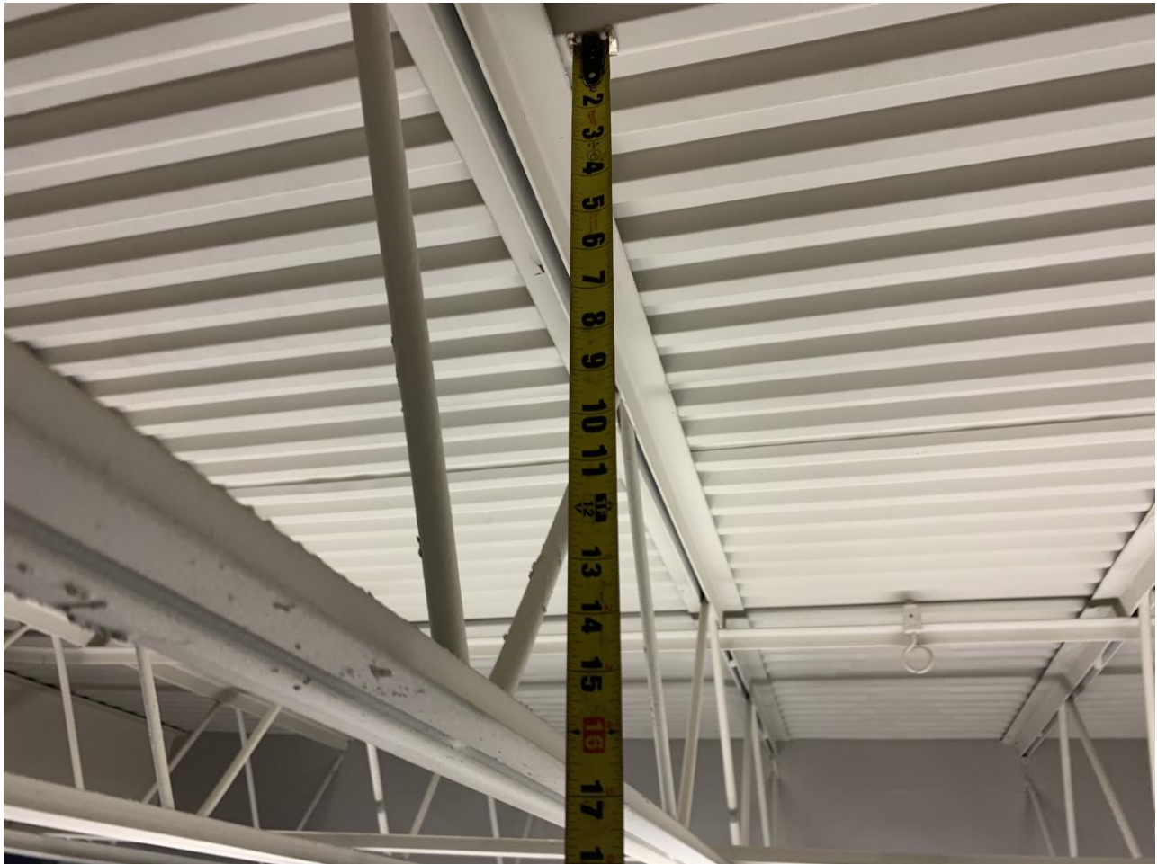
Photo 4: Typical depth of Joists noted during site visit
