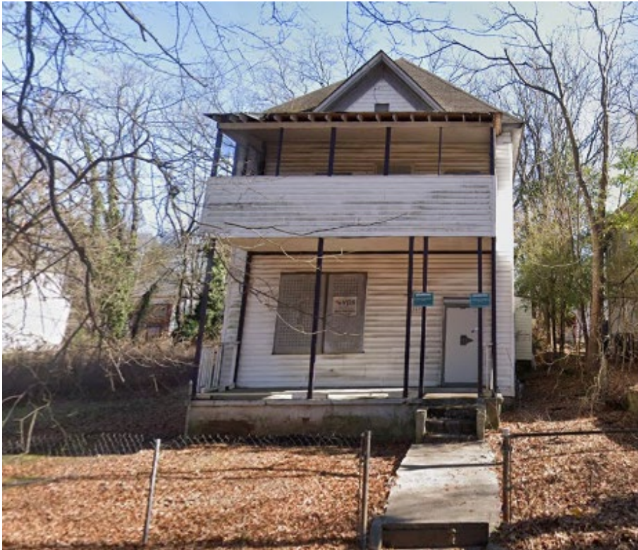
549 English Avenue Existing Condition
