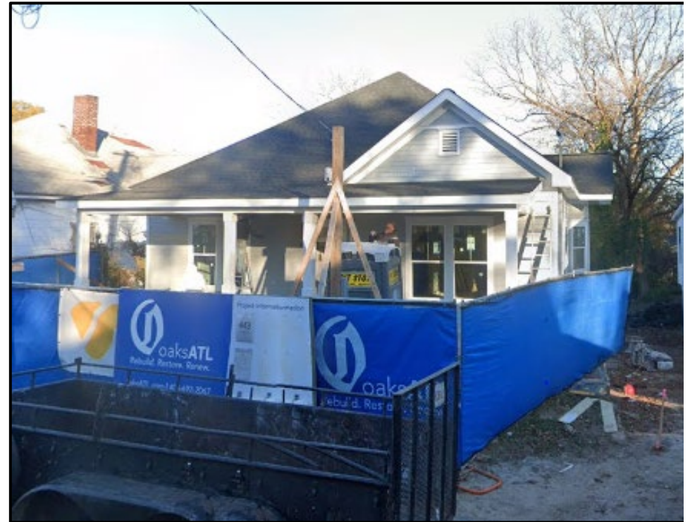
443 James P. Brawley Active Renovation
