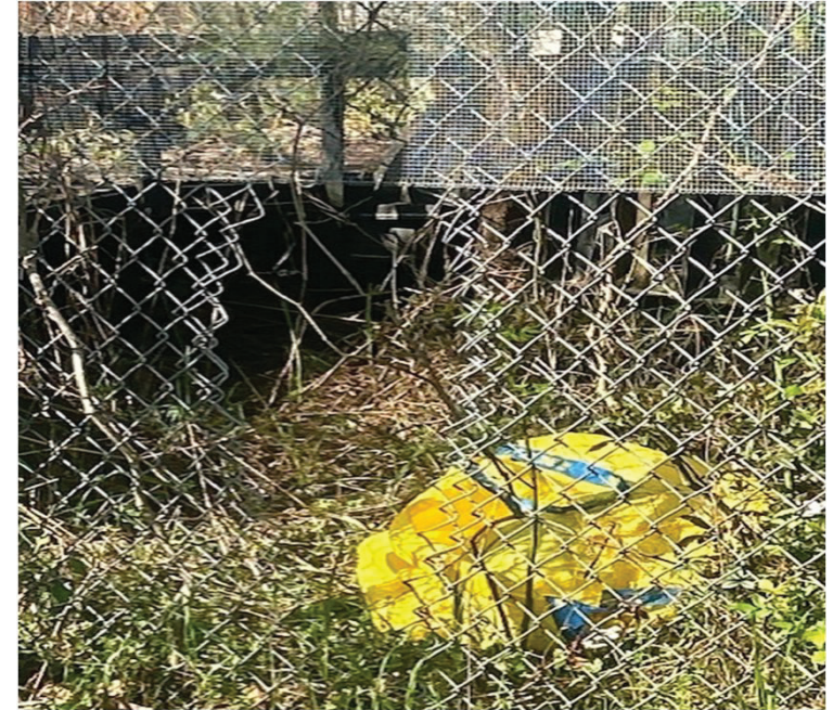
Fence Line Breach
