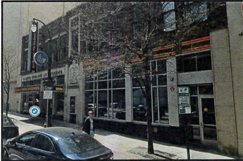
Existing Site Photos
