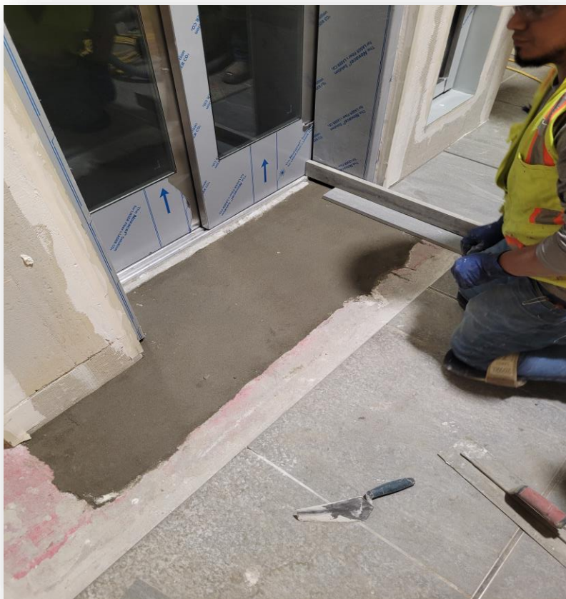
New Tile Installation
