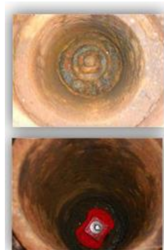
Before and After Op Nut Repair
