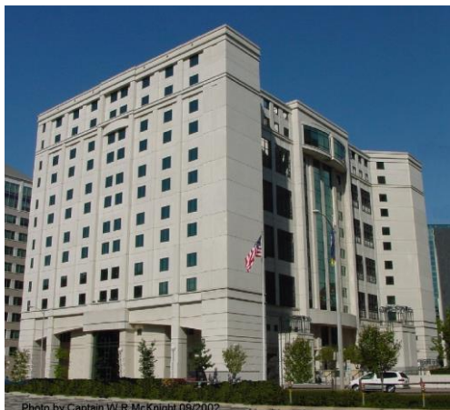
Arlington Detention Center
