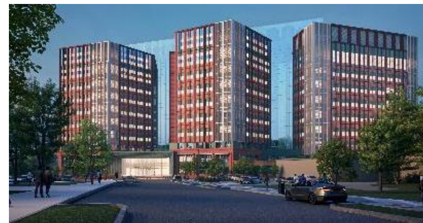
Confidential Urban Jail In Progress
