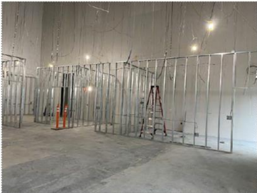
DREAM Office area wall framing
