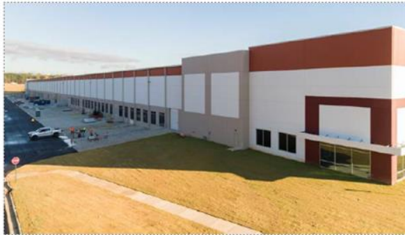
Building south facade
