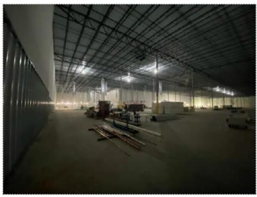
IT Warehouse looking at Police area
