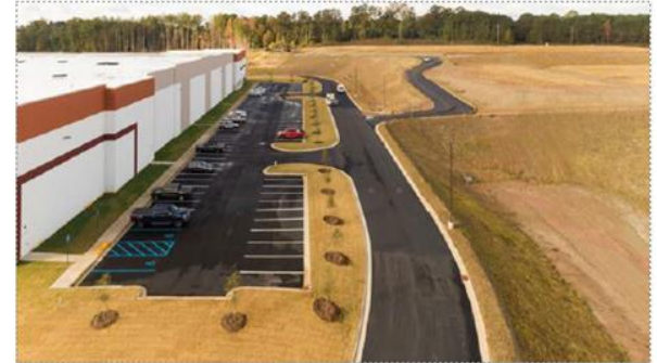
Building north facade
