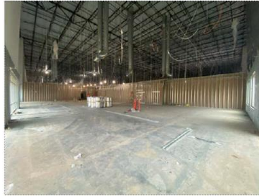
IT Office area demising wall
