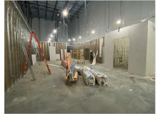
EMA Office Area wall framing
