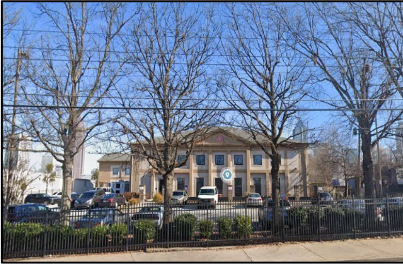
Existing administrative offices
