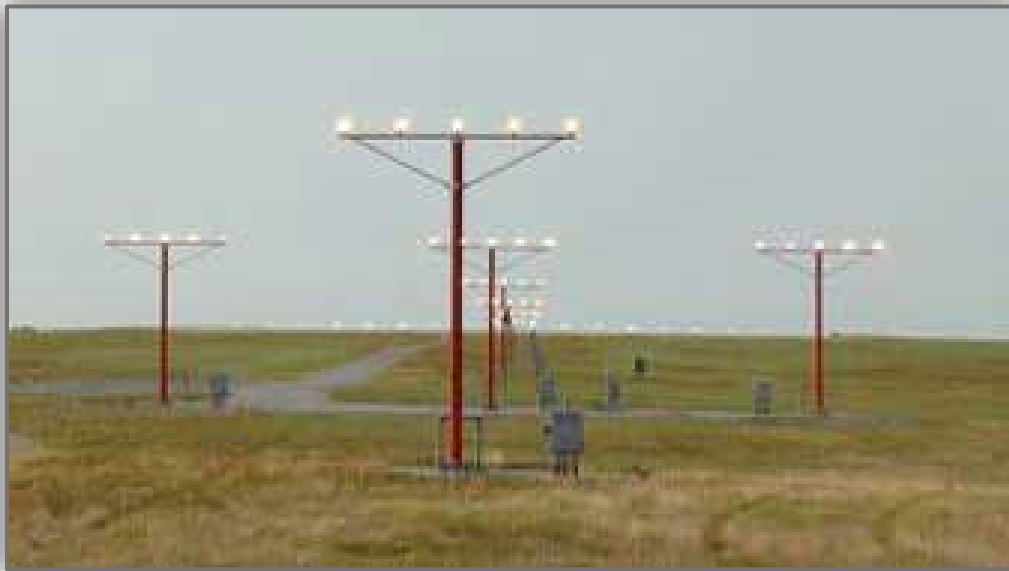
FAA, Lighting System – Medium Approach Light System with Runway Alignment Indicator Lights (MALSR), 2019.
